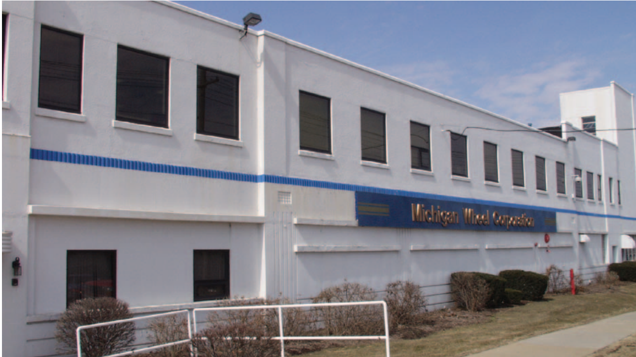
Michigan Wheel Corporation - Headquarters
