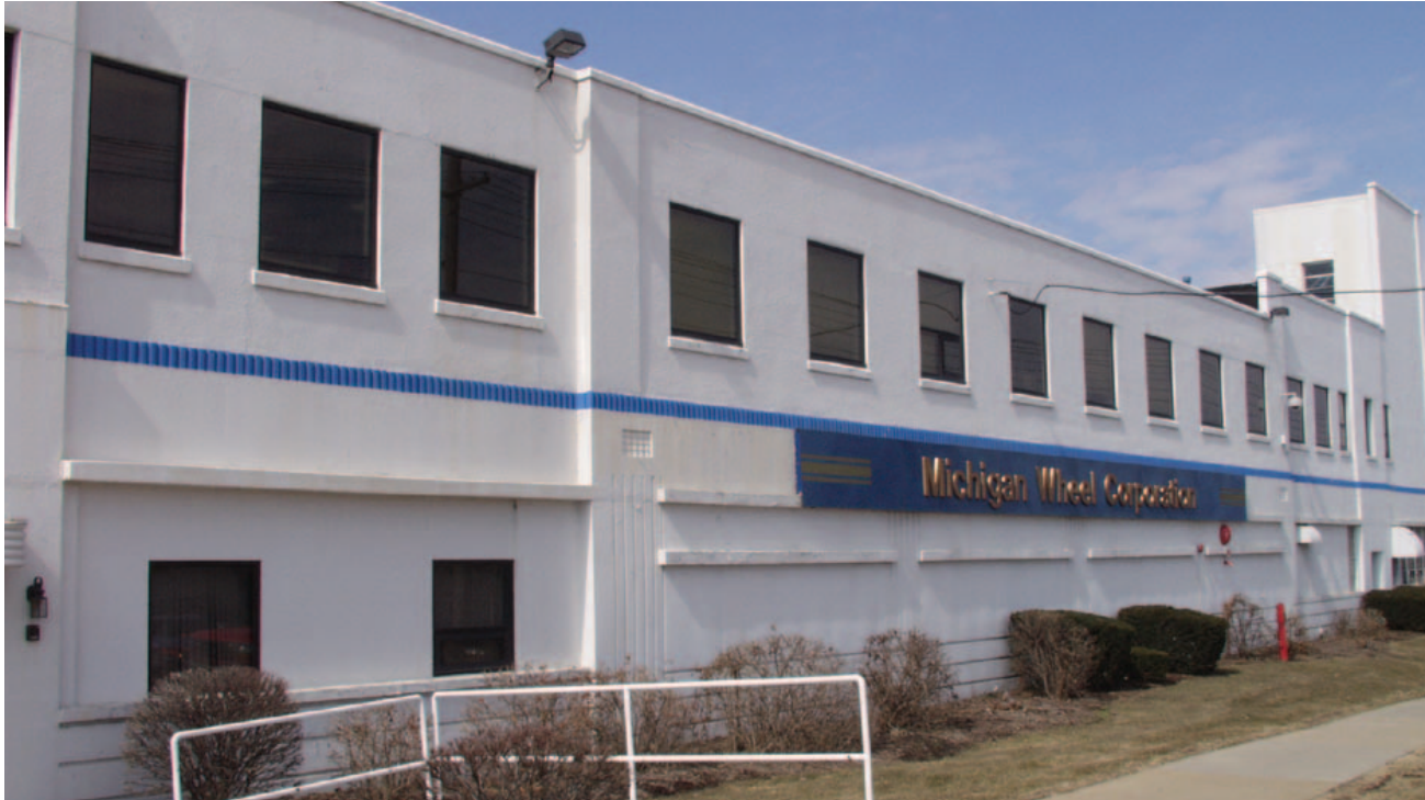
Michigan Wheel Corporation - Headquarters
