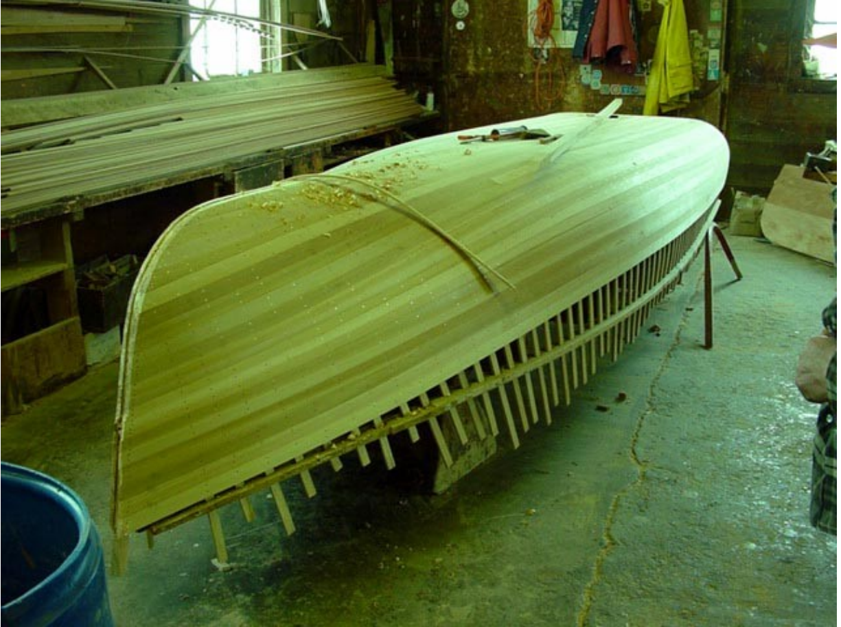
3)French River under construction
